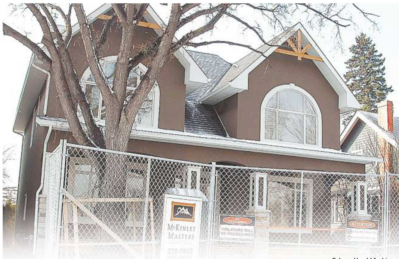
A new house by McKinley Masters Custom Homes arises on the site of a demolished home in Calgary. Calgary Herald Archive
