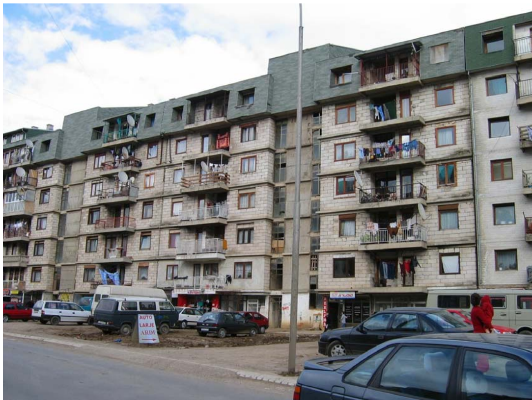
Multi-apartment housing built in the early 1990s in Pristina with visible signs of deterioration
