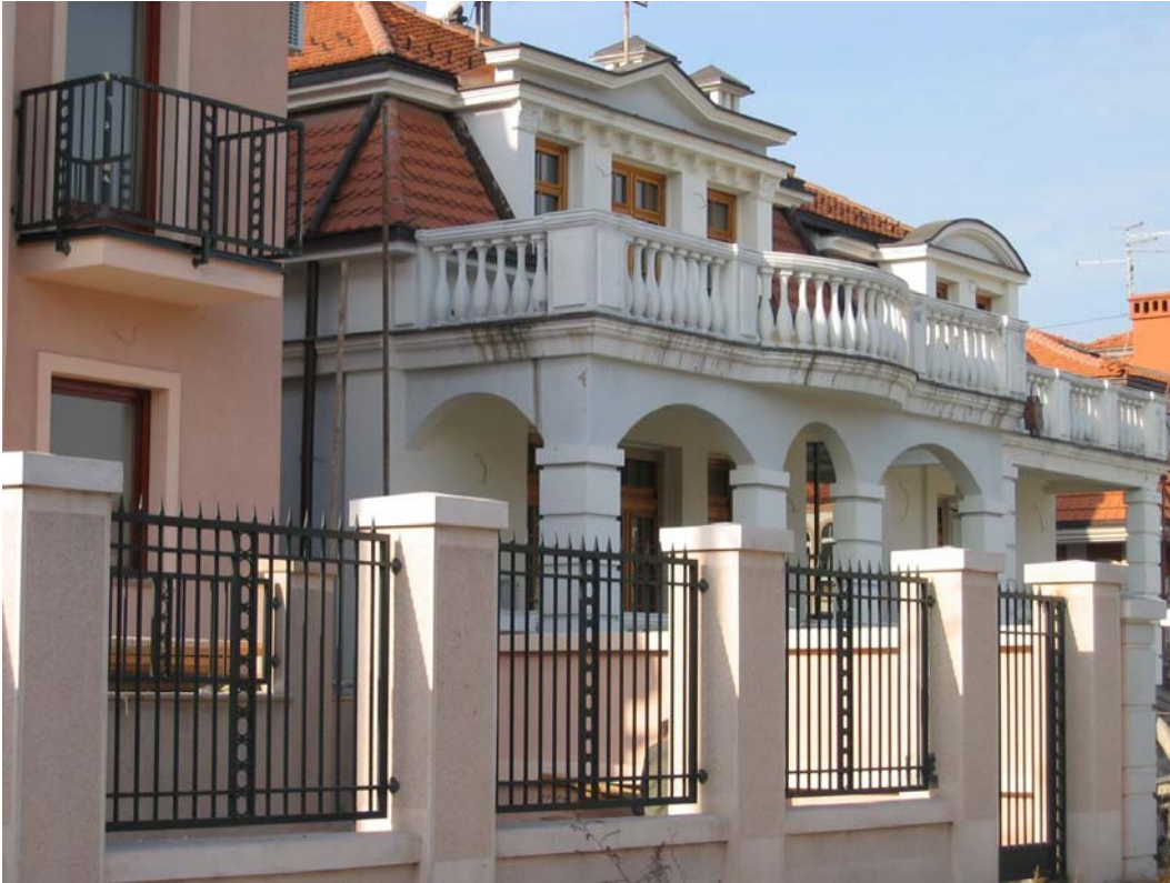
Illegally constructed housing in Belgrade
