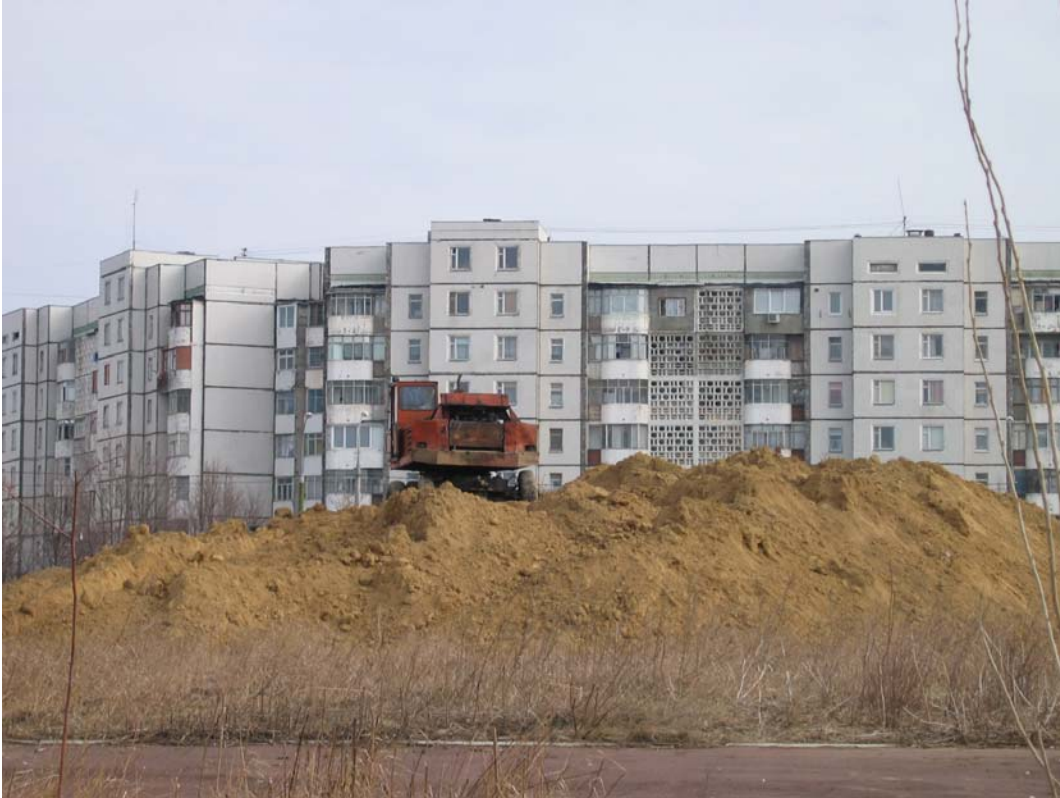
Chisinau: Multi-apartment buildings are often of poor quality with substantial investment needs.
