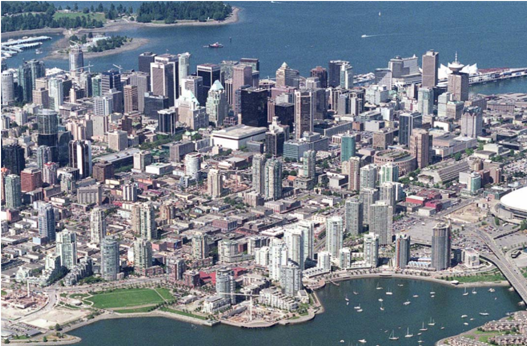
Growth in Greater Vancouver is managed through a regional sustainable development strategy which steers development into designated town centres. Extensive public consultation is an integral part of Vancouver's CityPlan and Community Visions process to ensure adequate representation of different social groups.
